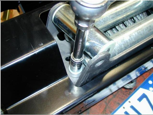
53. Tighten all bolts using socket and extension.
